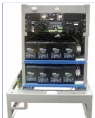
FXM Outdoor UPS and Lead Crystal® batteries fitted into sub-frame ready for integration into a standard Siemens controller cabinet
