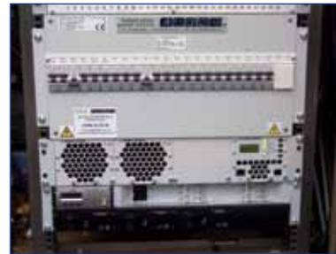
A typical Harland ProtectUPS® - T upgraded UPS system incorporating new style modular inverters and DC rectifiers
