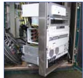
A typical 3 hour autonomy new Lead Crystal® battery arrangement fitted on easy slide shelves and swing frame UPS for ease of service and maintenance
