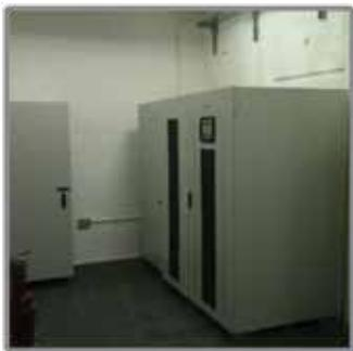
Within a short period of the above installation HS UPS was asked to supply 2 x Riello MHT400 KVA UPS's. Due to the tight space restraints, for this installation, Harland Simon provided open battery racks each fitted with 3 strings of batteries.
